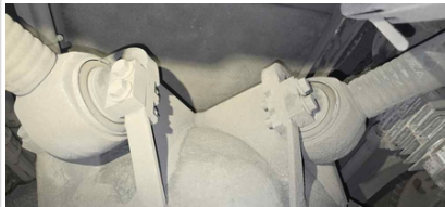
BUSHING STARTING TO CRACK
